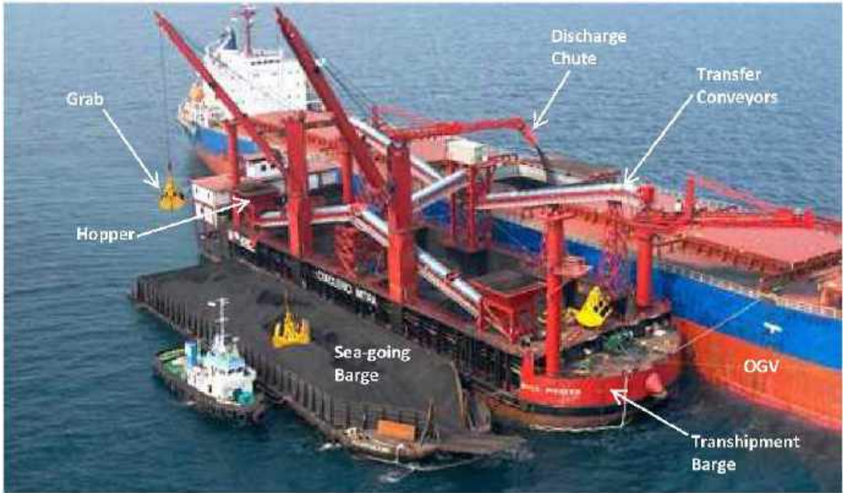
Figure 14 Example of a Typical Transshipment Facility
